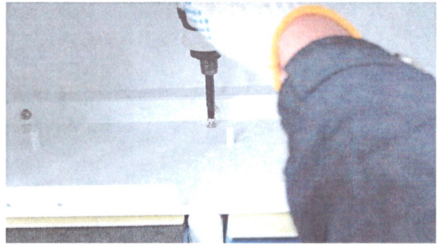
6. Use M4*10 screws to fasten the top panel
